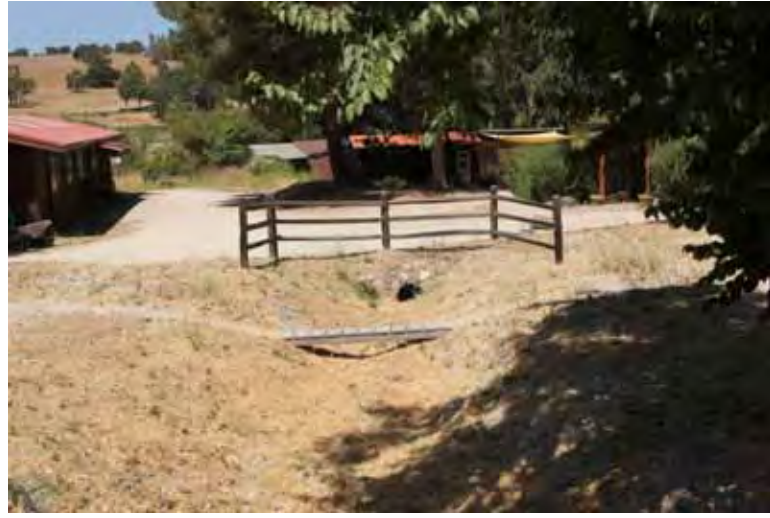
Erosion and flood danger
